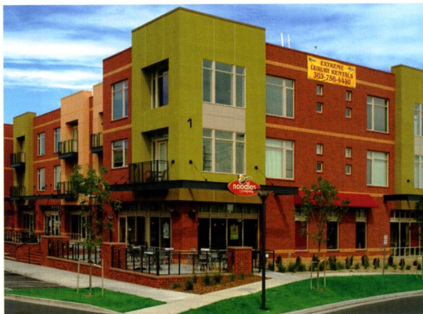
Project designers wanted a look that was sharp and trendy for the younger generation, yet something that conveyed a sense of high quality and solid construction for the Baby Boomers.
